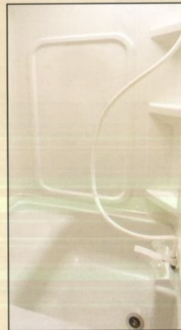
A one-piece molded tub surround helps protect shower walls and allows for easy cleaning.
