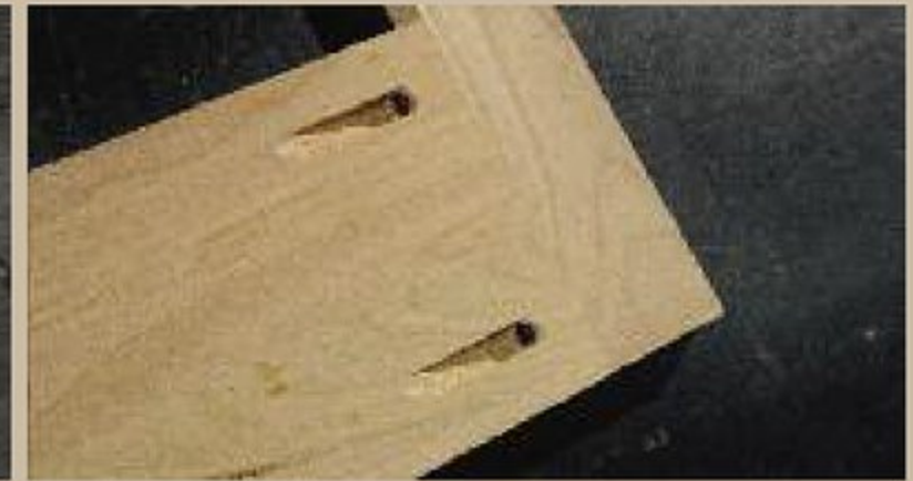
Pocket screws for structural integrity
