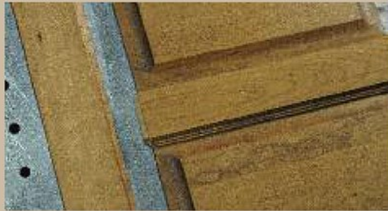
Raised panel door detail
