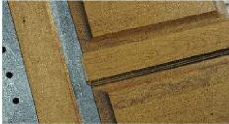
Raised panel door detail
