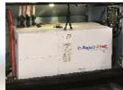
Aqua-Hot hydronic heating system
