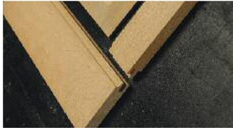
Dovetail construction
