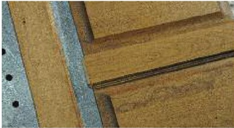
Raised panel door detail
