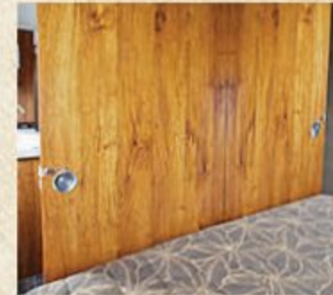
POCKET DOORS IN BEDROOM
