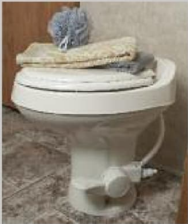
Toilet with foot pedal and "power flush" jets
