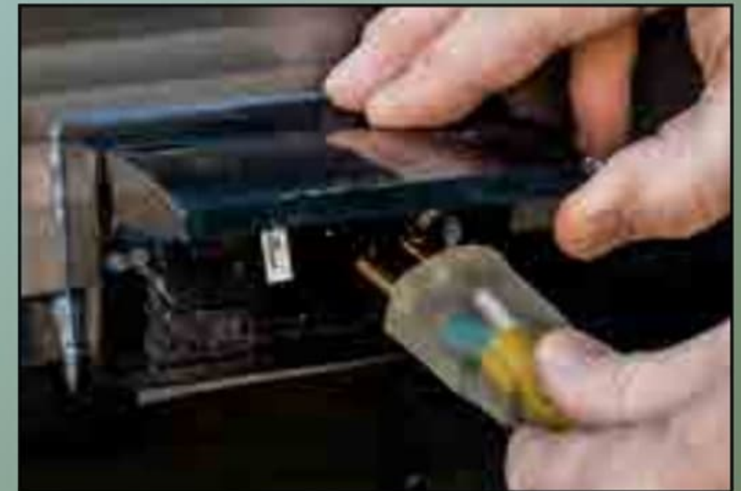
Convenient Outside GFCI Protected and Covered Outlet.
