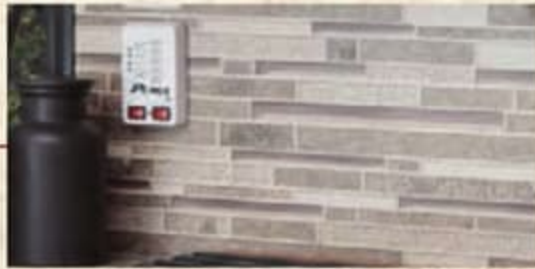
Decorative backsplash with monitor panel that indicates battery strength, tank capacity and water pump details.
