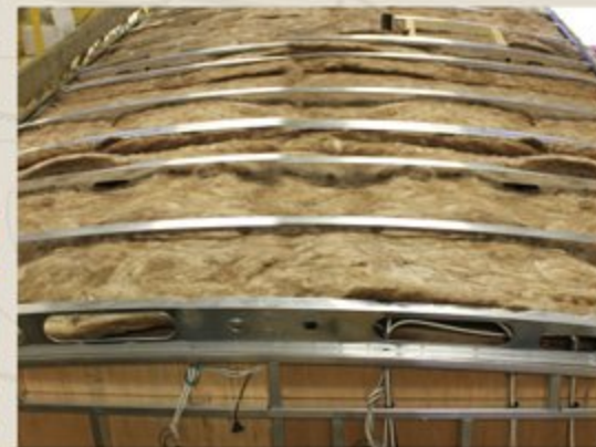
Steel truss roof system
