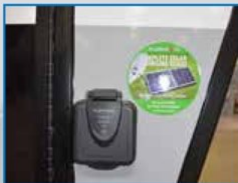
SOLAR PREP AND WIRING
