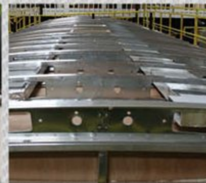
Walkable steel truss roof system
