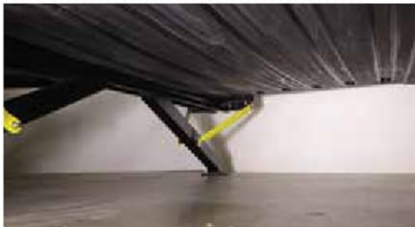
Heat is routed into individually insulated holding tanks to keep them, the valves and PEX lines warm.
