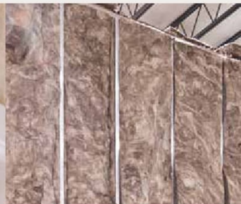
R-16 residential insulation completely surrounds all of our walls and slides. Best insulation in the industry and eco-friendly!
