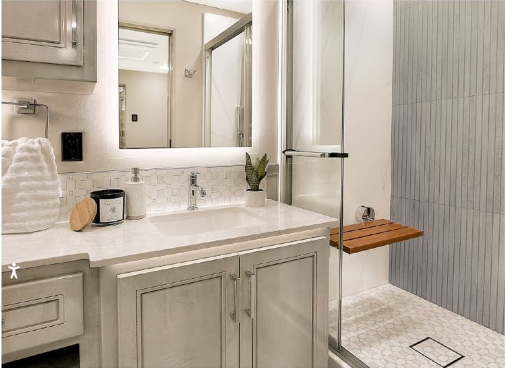
Cape Cod Cabinetry // Haven Interior Décor // The bathroom features a solid surface shower with an accent tile wall, floor inlay, an integrated niche and a sliding glass door.
